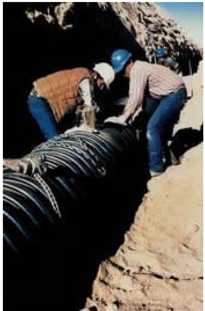
Assembling a Spirolite ® Joint
