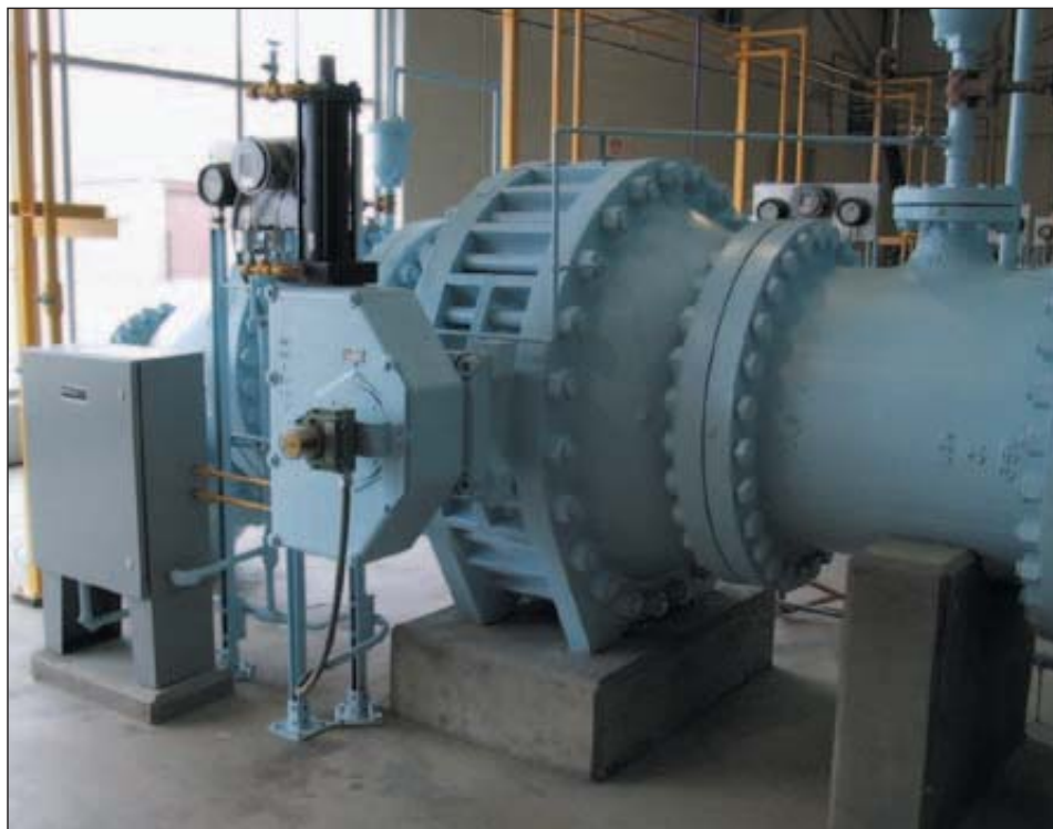
Rubber Seated Ball Valve Installation
