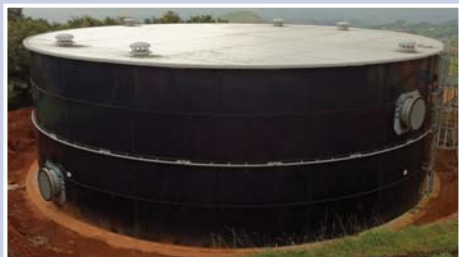
Trough Deck Roof
