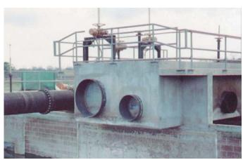
Coplastix Weir Sluice Gate mounted over circular holes
