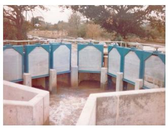
Coplastix Channel Mounted Sluice Gates
